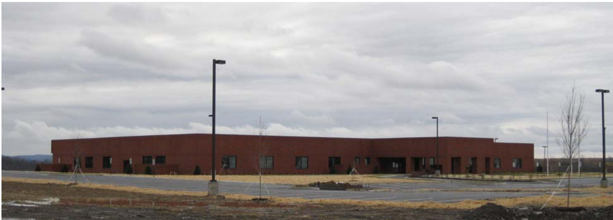
Photo 2. The Sykes Enterprises building at the Southern Gap Development Area in Buchanan County (see Photo 1), in winter prior to initiating operations. Because the site was compacted thoroughly and effectively during reclamation operations, the firm was able to install modern communications equipment that is sensitive to ground movement, as on a natural site.
